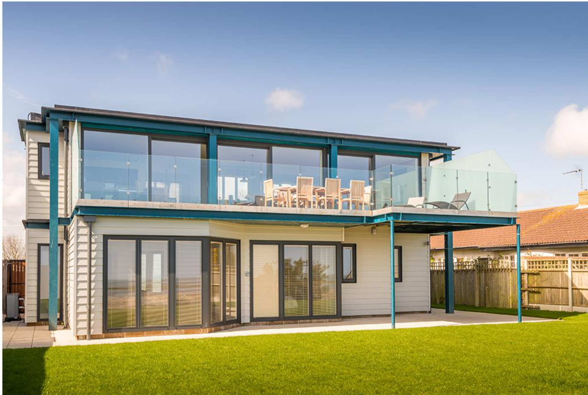
Eva's Lookout is designed in an unusual 'upside down' style with the living room occupying the second floor
